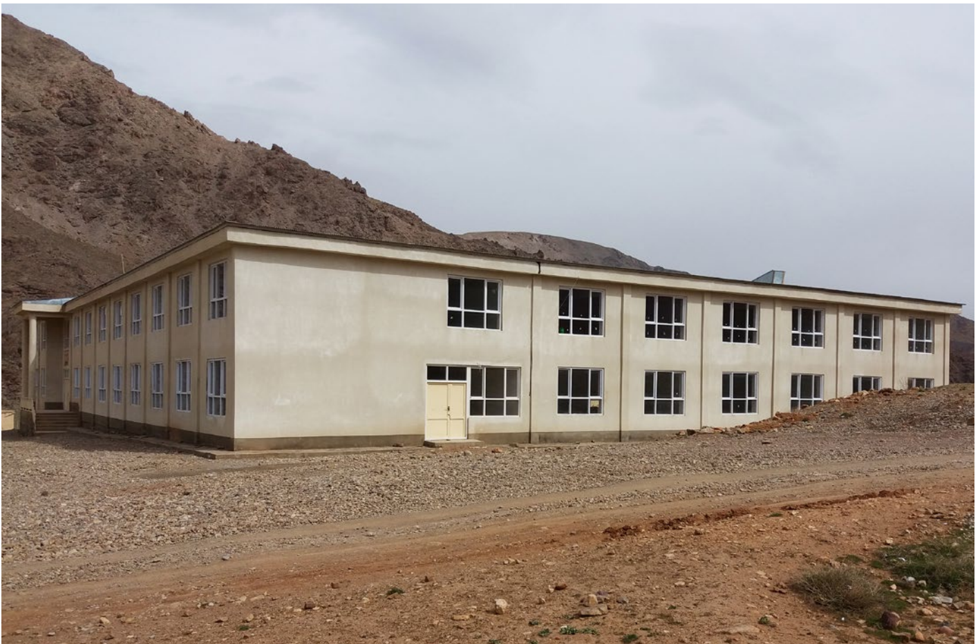
Responding to acute educational needs in the province, this school was newly constructed in Malistan district, Ghazni province. © IOM 2020
